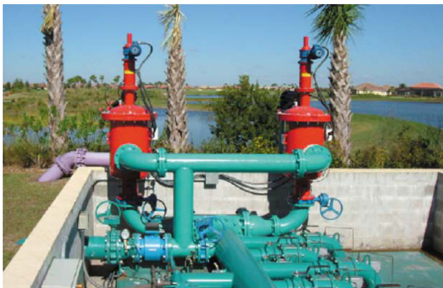
Golf course irrigation. 700 m 3 /h, 200µm. Tampa, USA
