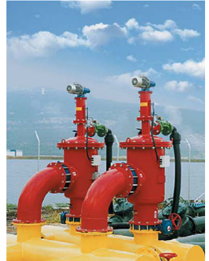
Reservoir water for irrigation. 1000 m 3 /h, 100µm. Kfar Hasidim, Israel
