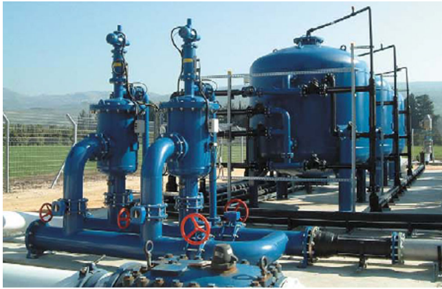
Pre-filtration to DWP. 375m 3 /h, 50µm. Dan river, Israel
