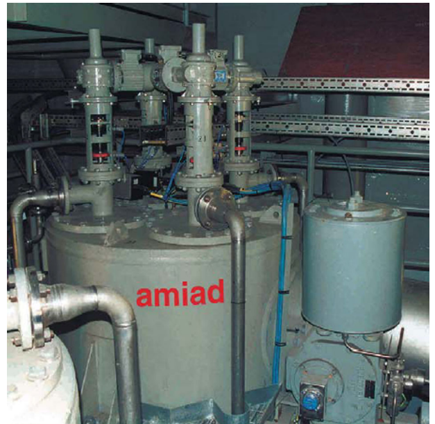
Injection water. 2000 m 3 /h, 50µm. North Sea Platform
