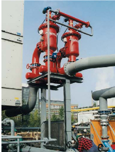
Cooling water in chemical plant. 460 m 3 /h. Hamburg, Germany
