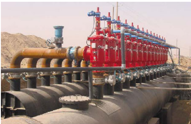
Drip irrigation, 9000 m 3 /h, 130µm. China
