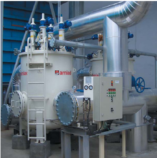
Industrial wastewater. 800 m 3 /h, 50µm. Electronic industry, Korea
