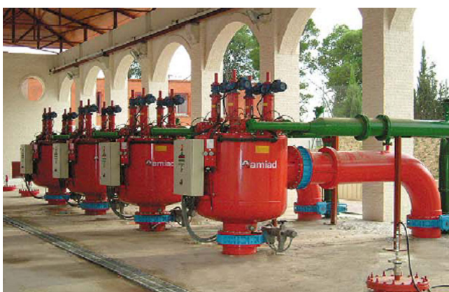
Drip irrigation, 8000 m 3 /h, 130µm, Helche Creviente, Spain
