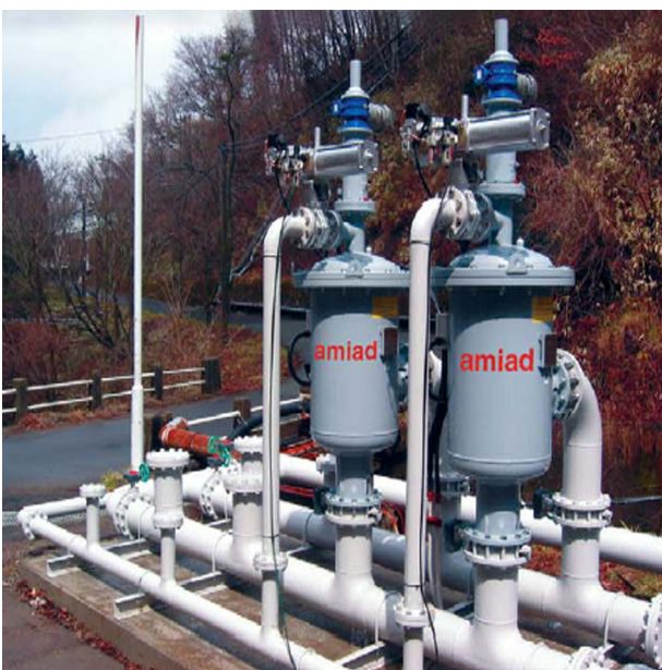
River water for hot spa. 170 m 3 /h, 25µm. Japan
