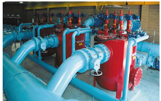
Recreation and irrigation water supply. 3400 m 3 /h, 80µm. Spanish Fork, USA
