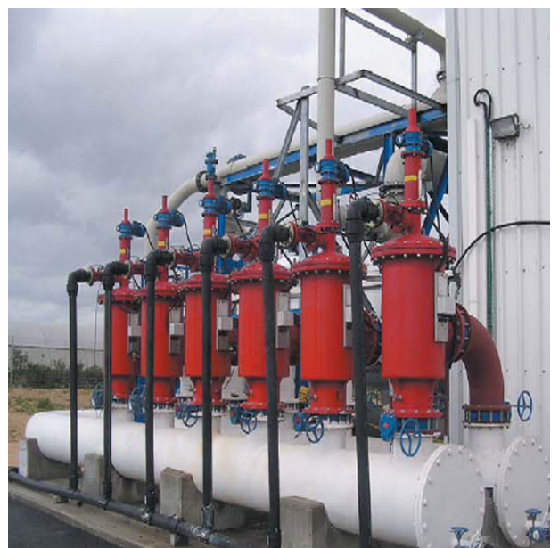
Pre-filtration to RO membranes. 1700 m 3 /h, 25µm. Desalination plant, Israel
