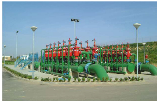
Drip irrigation of strawberries. 14,000 m 3 /h, 130µm. Spain
