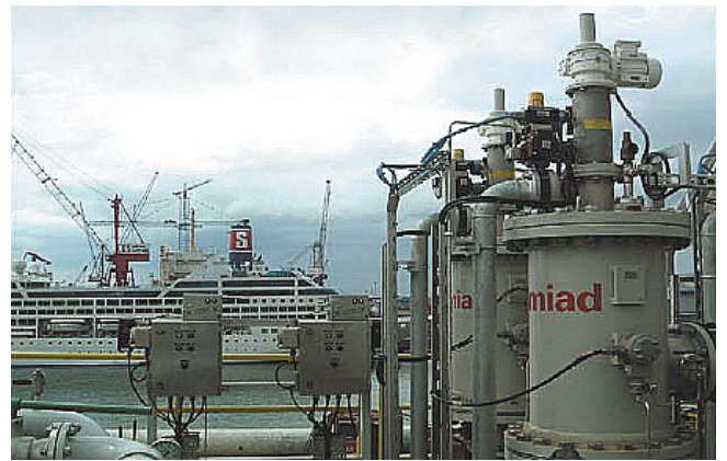
Injection water on board FPSO. 220m 3 /h, 25µm. West Africa
